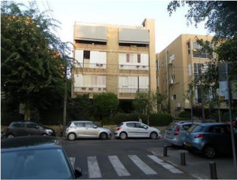
93, Sokolow Street, an ordinary colonnade apartment building opposite Amos Street
